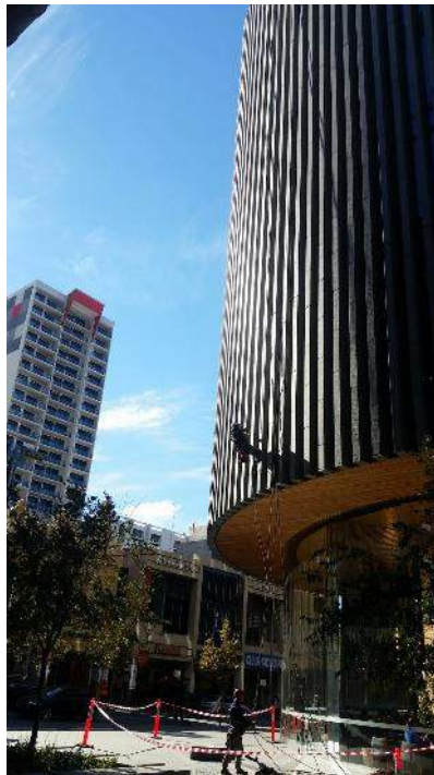
Rope Access Façade Inspection work on the City of Perth Library
