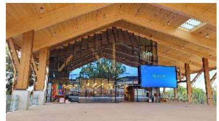
Murdoch University New Administration Building
